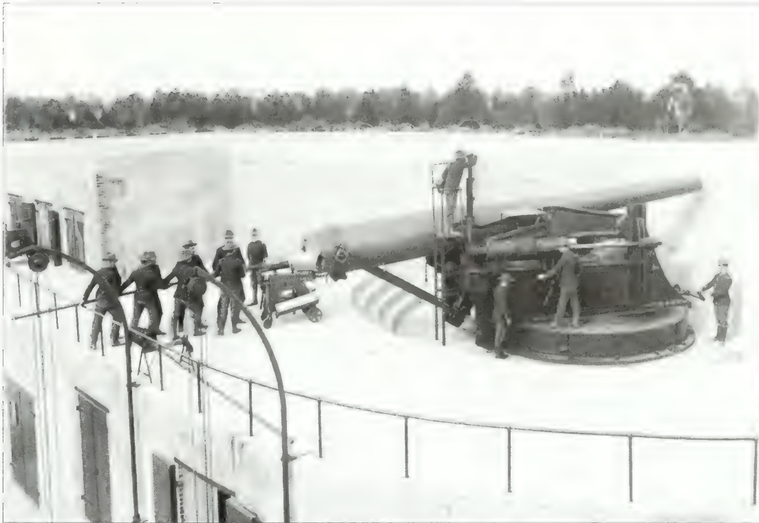
Figure 5.63. Battery Granger, circa 1900. Note the growth of woody vegetation beyond the limits of the engineered slopes. Great effort was made to disturb as little pre-existing vegetation in front of the battery as possible in order to conceal the structure from enemy fire (GATE 7778).
